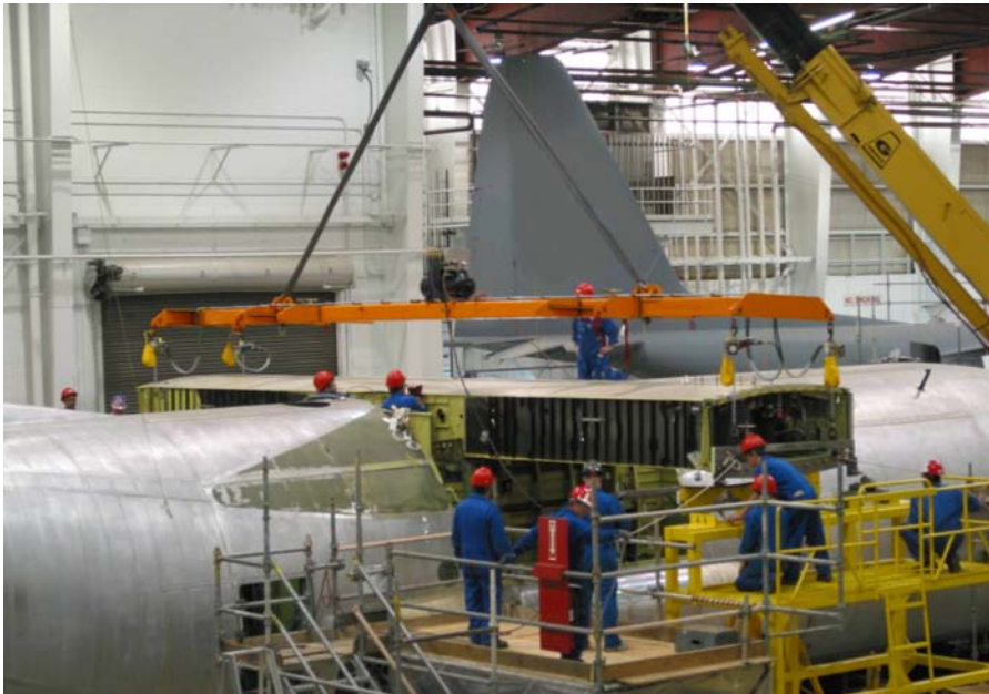
Figure A-3 Positioning a C-130 Centre Wing
