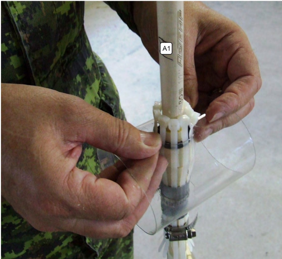
Figure 28-A Sliding the Spring over the Cable Ties
